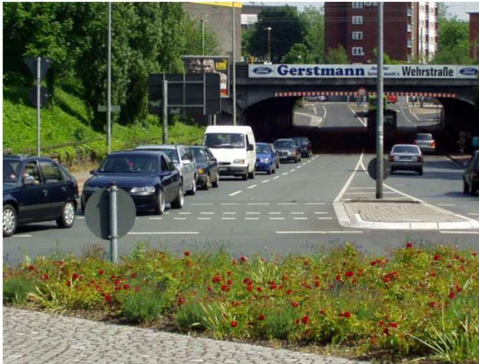
Fig. 9: Typical driver behavior at a compact two-lane roundabout: unused left lane on a two-lane entry
